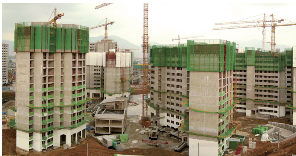
Above: New apartments under construction in Seoul.
